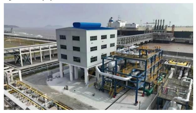
This Power Generation Unit with a 4,000kW turbine that uses LNG cold energy for generating electricity was additionally installed in the existing LNG receiving terminal where IPC, as a member of consortium contractor for the project, built three 165,000 kiloliter LNG tanks in 2009.
